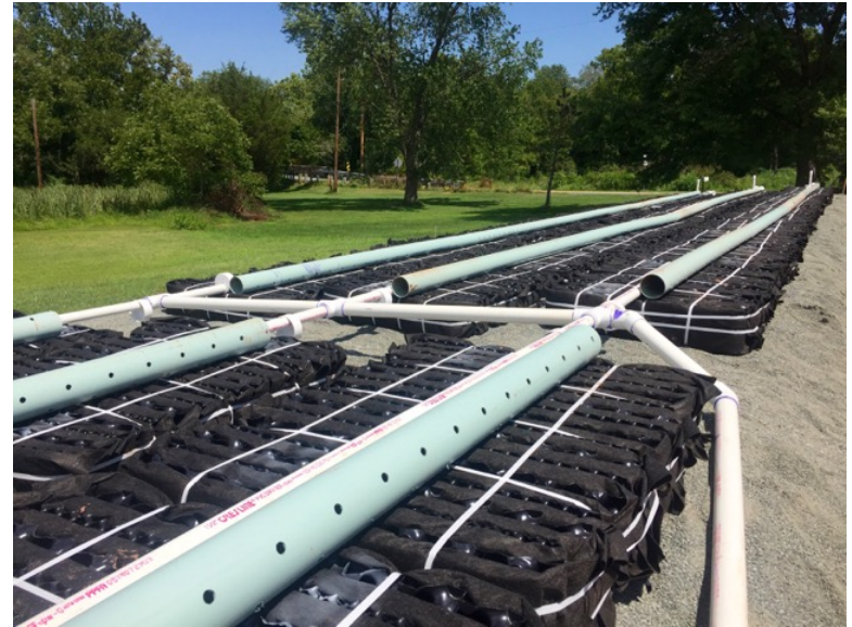
4" PERFORATED PIPE (SDR 35 OR BETTER)
