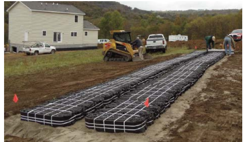
Eljen B43 modules placed end-to-end in a bed configuration.
